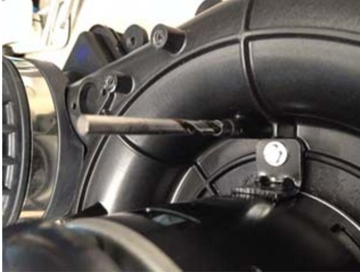
7. Re-install the inducer assembly. Attach with 5 screws, connect inducer motor wire harness and connect vent pipe.
