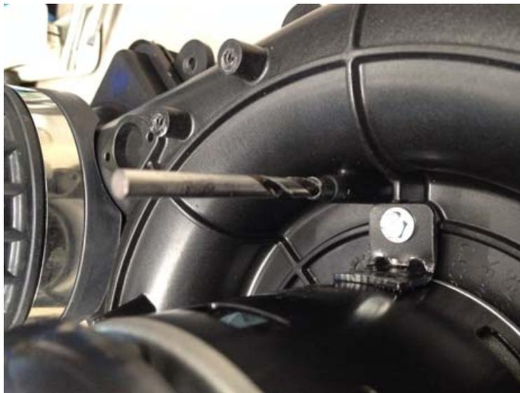
6. Use the 3/16" drill bit to enlarge the port. Do not exceed the depth of 1 1/2"
