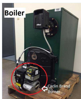
Carlin Brand Burner on Boiler
