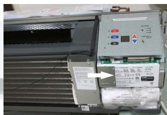
Model and serial numbers can be found by lifting the unit's front cover.
